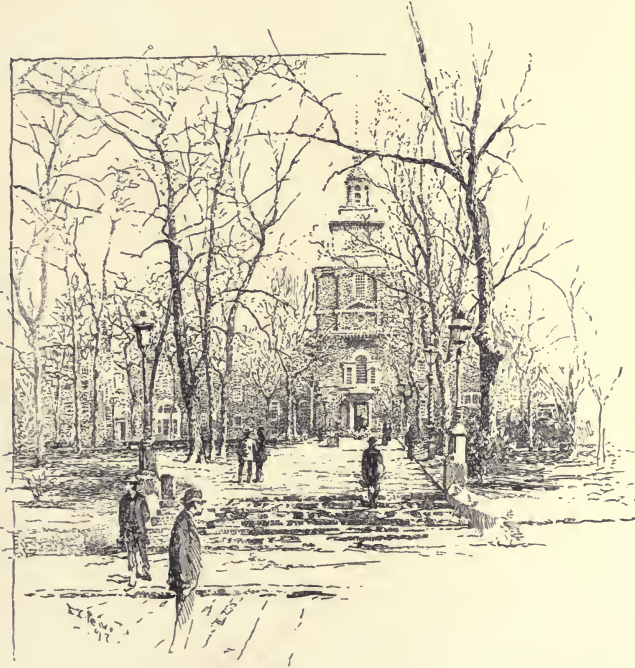
VIEW OF INDEPENDENCE HALL FROM THE PARK SIDE.
